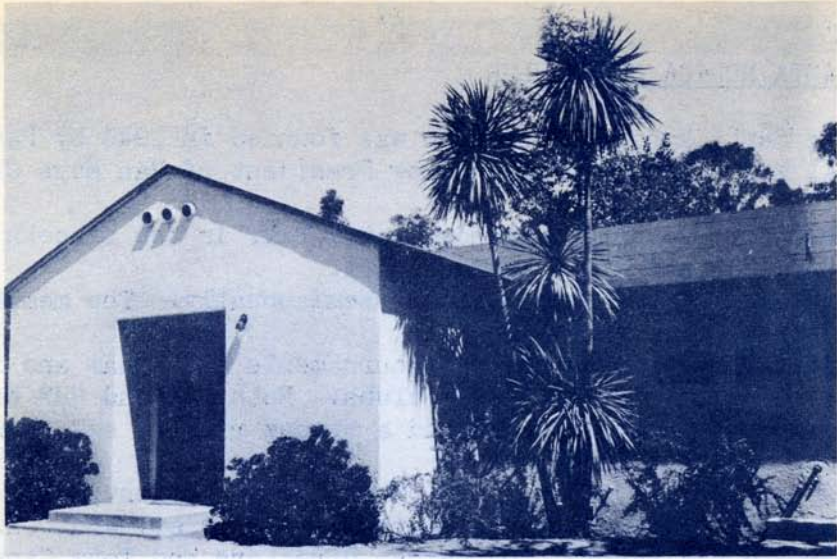
Valley Chess Clubhouse, North Hollywood Park
